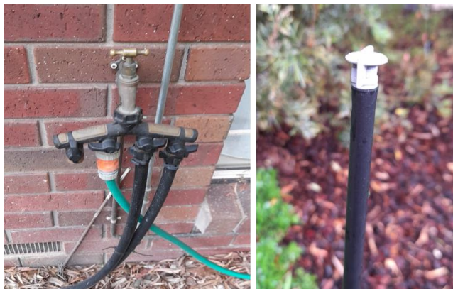
Manual watering system with sprinkler heads (Photo: Paul Birch)
